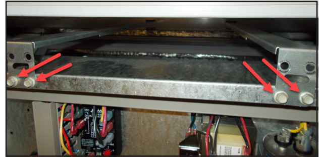
FIGURE 6 Remove Four Screws
