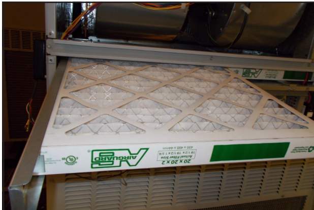
FIGURE 10 Install Left 2" Filter
