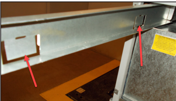
FIGURE 5 Bend Filter Tabs Down
