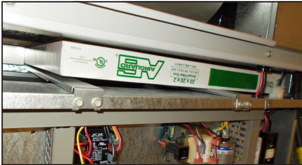
FIGURE 10 Install Left 2" Filter
