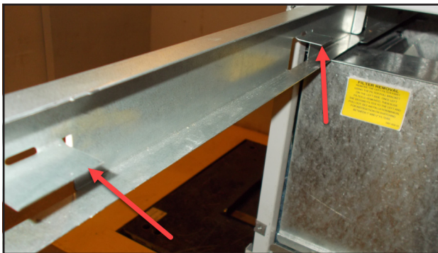
FIGURE 4 Filter Tabs in Up Position
