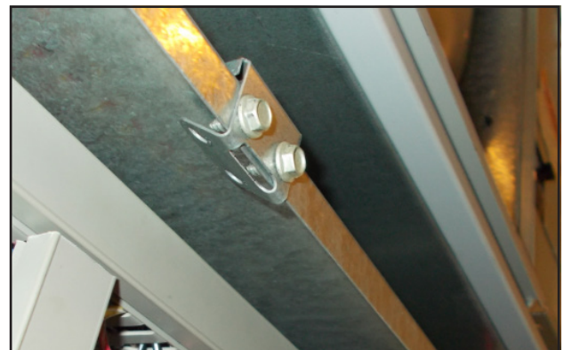
FIGURE 8 Re-Install Screws and Bend Tabs Up
