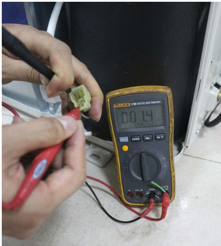
Fig. 63 – Test the voltage
