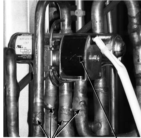
Brazed parts of 4-way valve R.V. coil
