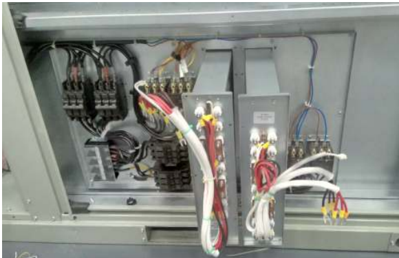
Figure 5. Electric heater aligned to screw holes
