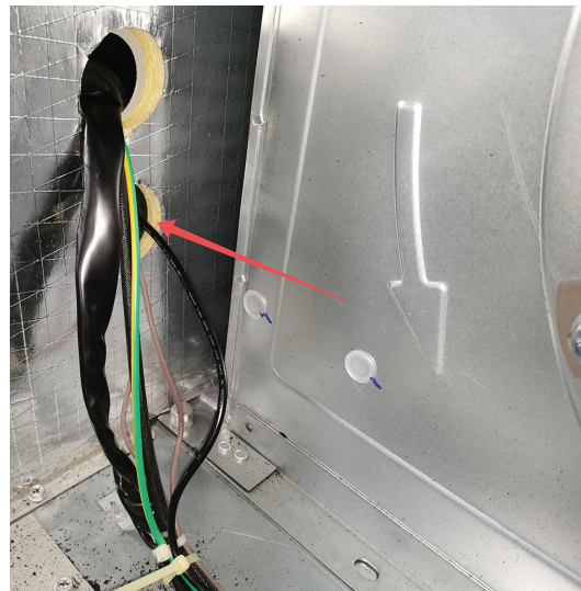
Figure 8. Supply fan blower section
